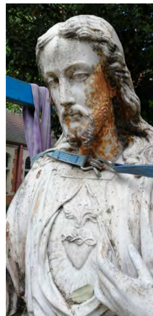
Small hoist used to carefully lift the statue from its plinth, 29 May 2024
