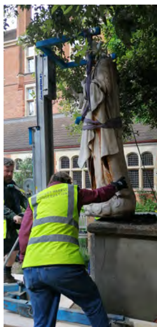
Small hoist used to carefully lift the statue from its plinth, 29 May 2024
