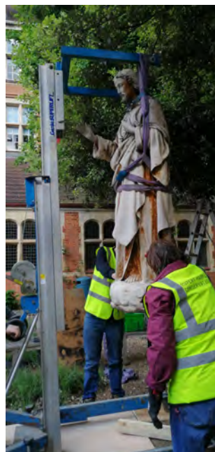
Small hoist used to carefully lift the statue from its plinth, 29 May 2024
